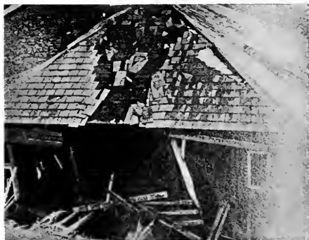
FIG. 140. Building wrecked by Explosion 145 yards away. Faversham, February 21, 1879
